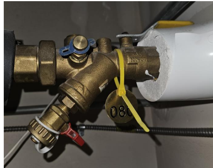
Typical strainer – clean out twice per year
